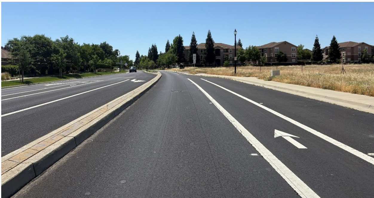
Image 3. Motorist's view of Hayden Parkway driving southbound with project site to the right
